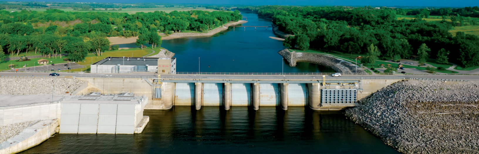
Completed upstream diaphragm wall, intake structure (left) near existing structures
