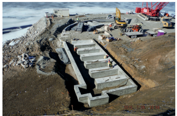
Guide wall for upstream diaphragm wall construction
